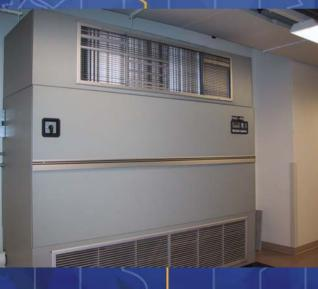
Traditional CRACs were not designed to cool High-Density Racks. They can actually cost 100-200% more to run than the server loads, and still not properly cool the racks.
